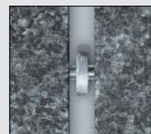
Appearance of joint with conventional dowel fixing
